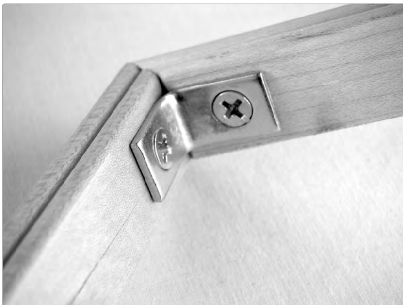
FIGURE 9-5: Detail of an inner frame corner brace
