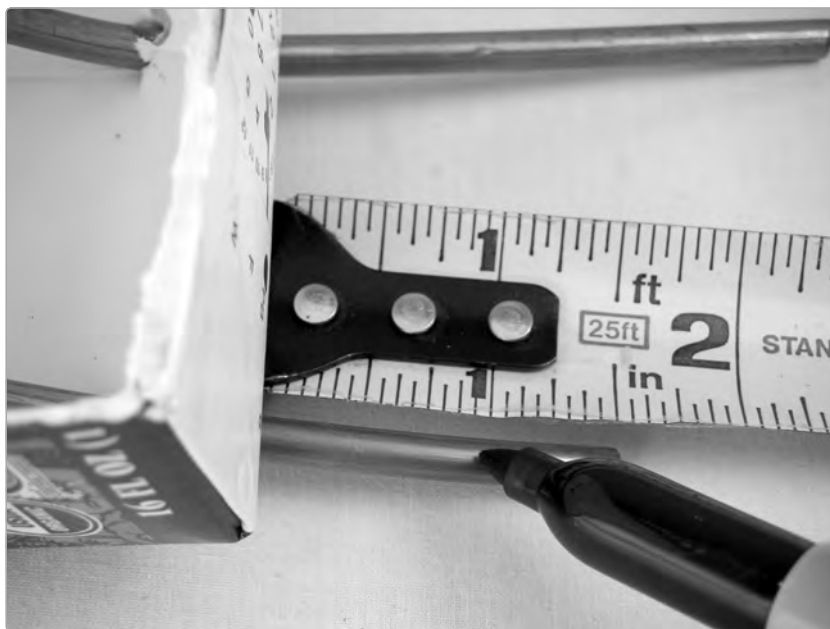
FIGURE 21-9: Marking the tailpipes for trimming
