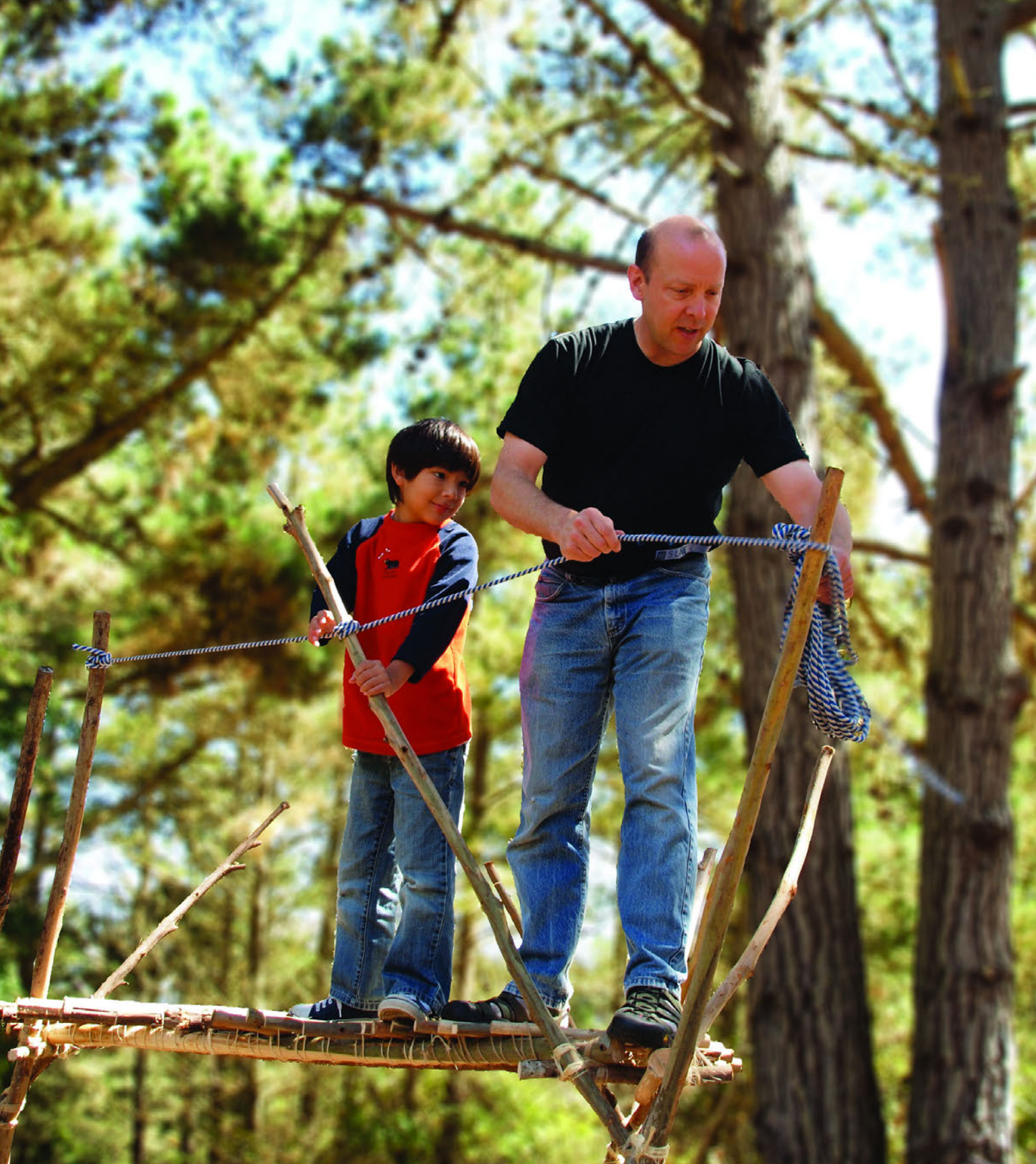
Figure 8-27 Not everything has to be sticks. We'll just finish it off with a heavier line here to make a railing.
