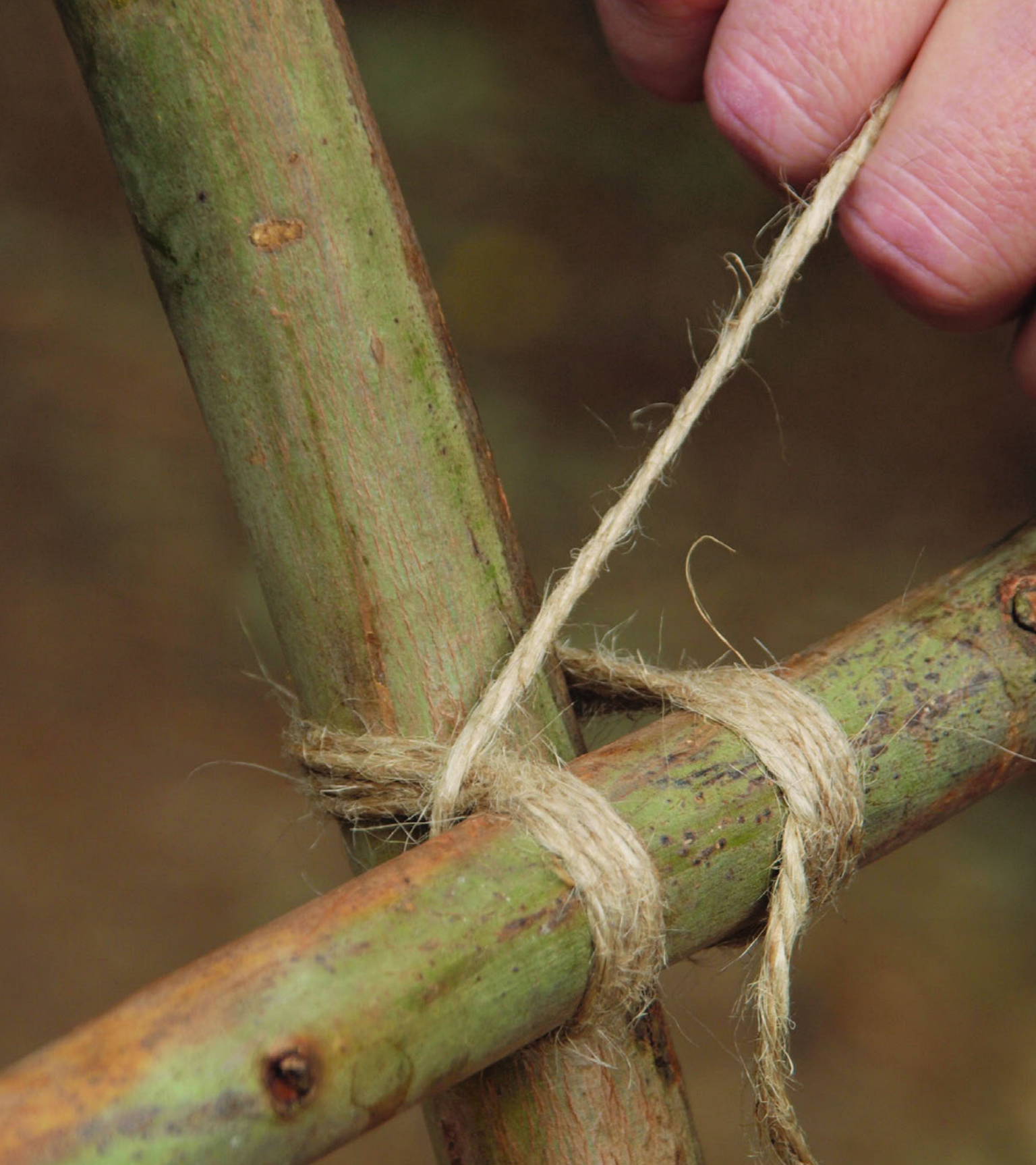
Figure 8-10 Then, to really crank up the tension, add crossing wraps.
