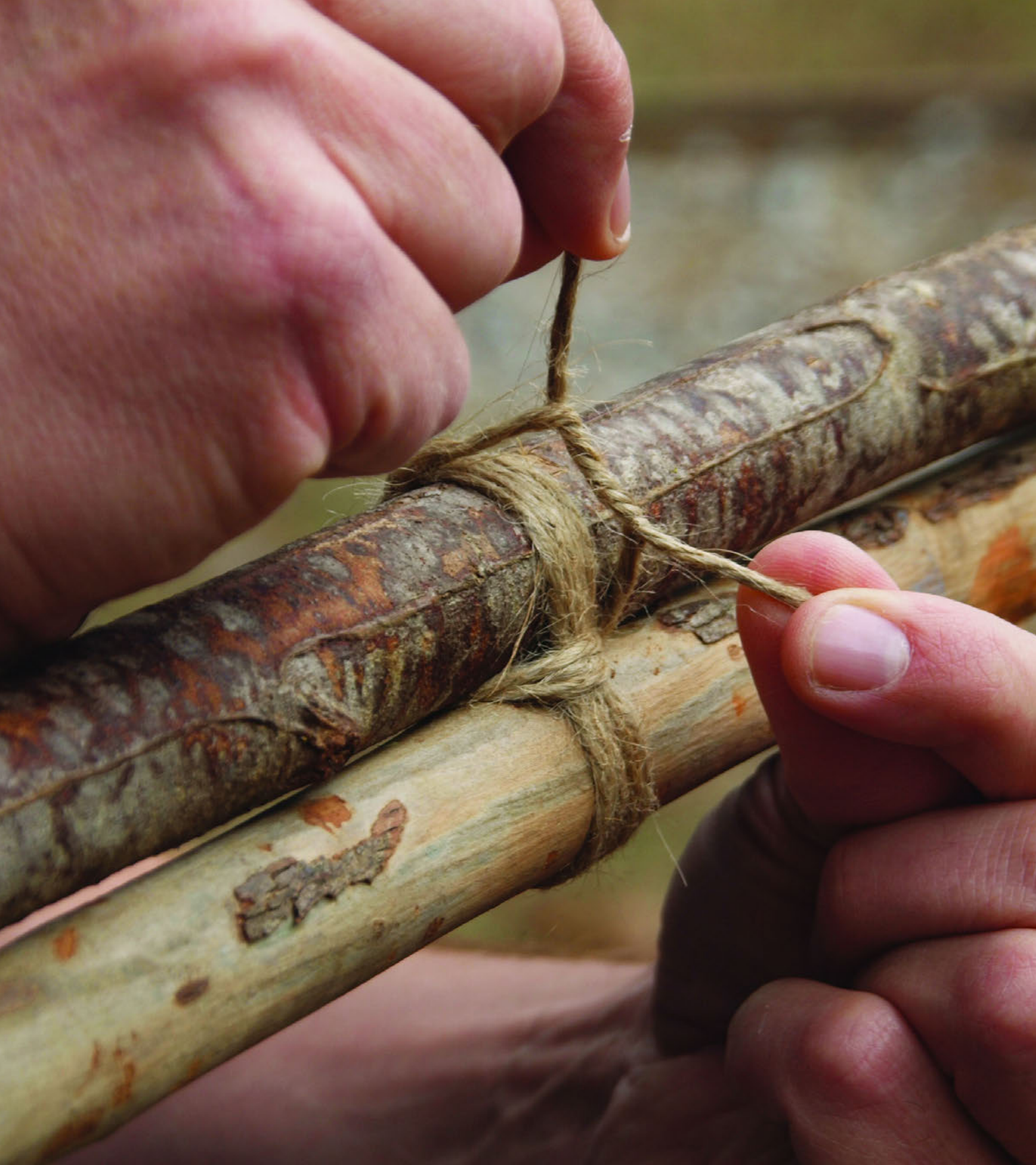
Figure 8-16 Add a few loops across the lashing to tighten it up nicely.
