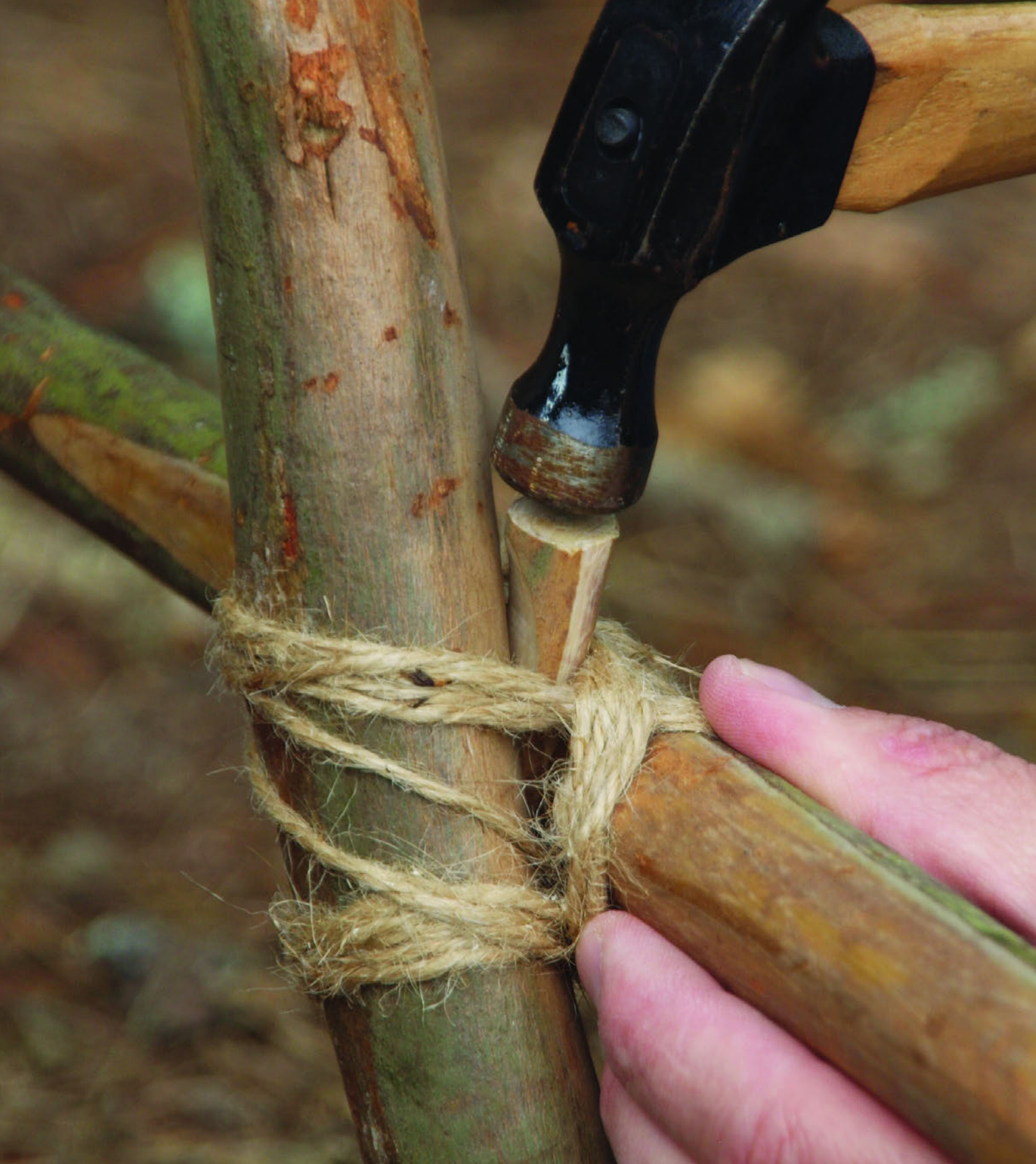
Figure 8-14 So if one joint gets loose, you can whittle a wedge and pound it under the line to tighten it.
