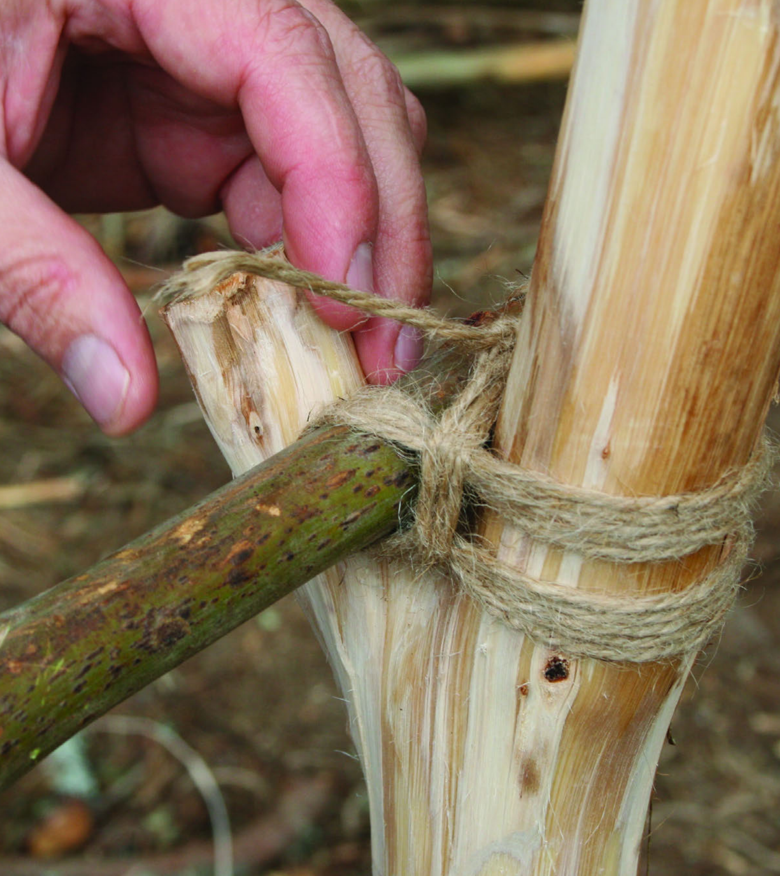
Figure 8-23 A natural fork can add strength to your construction. And you only have to lash to the strongest side; gravity does the rest.
