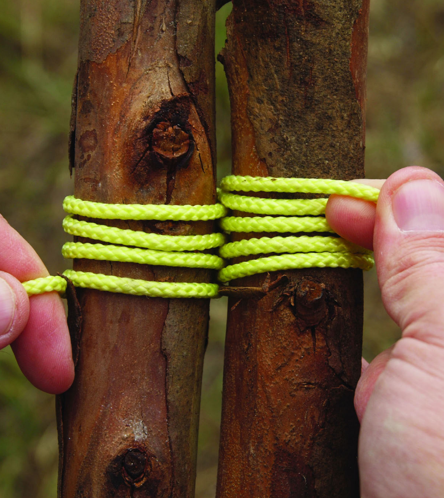
Figure 8-20 A secure, flexible connection is made by running the lashing between the sticks.
