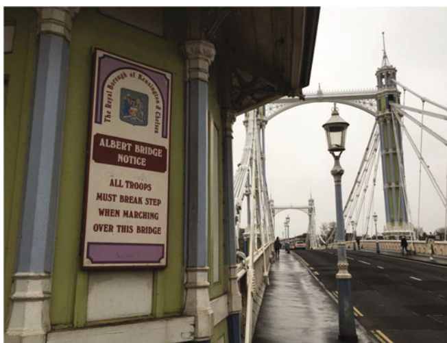
Figure 10.13. The Albert Bridge in London.
